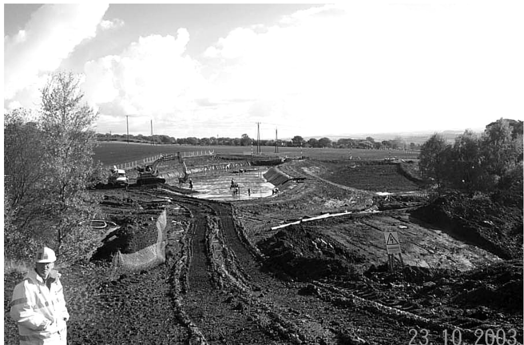
Figure 4.4: Earthworks for the full-scale treatment system at Bowden Close. In the background are the two RAPS lagoons. Only RAPS lagoon No 1 (to the left) has an artificial High Density Polyethylene (HDPE) liner.
