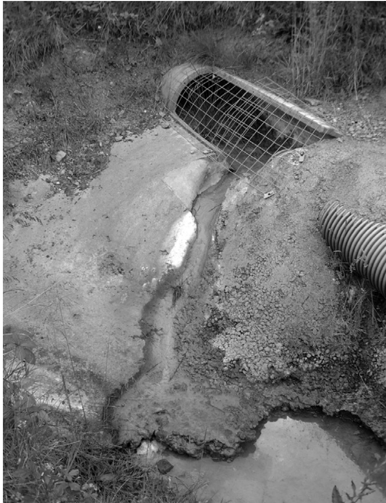
Figure 2.3: Seepage from the water gate of Harvey Drift is captured and diverted into No 1 discharge pipeline.
