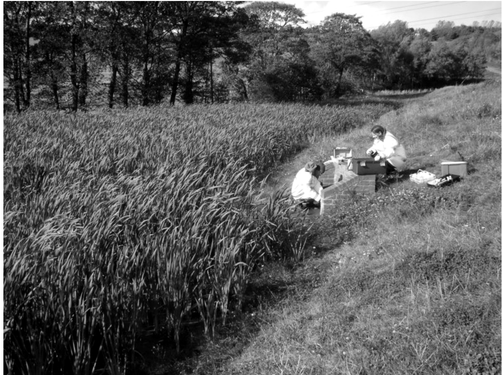
Figure 4.5: The aerobic polishing wetland of the full-scale system was planted with mature reeds in summer 2004.
