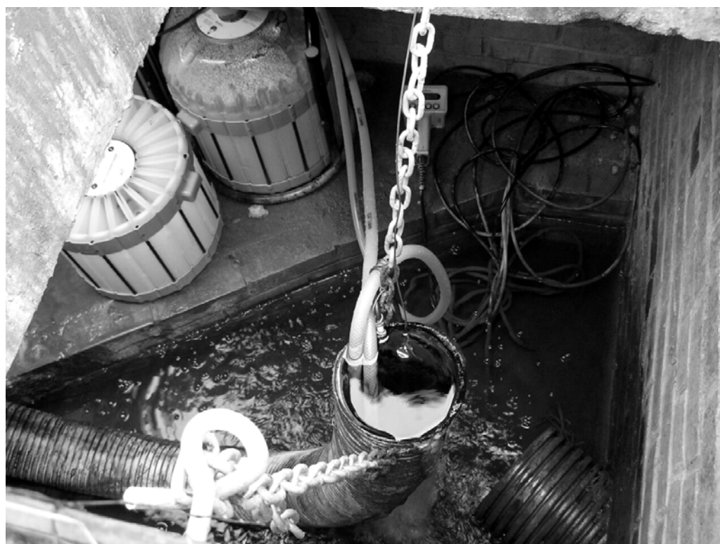
Figure 4.8: Each RAPS outlet is housed in locked chambers which can accommodate auto-samplers and monitoring sondes. The pipework ends in a flexible hose suspended on chains controlling the hydraulic gradient across the RAPS.
