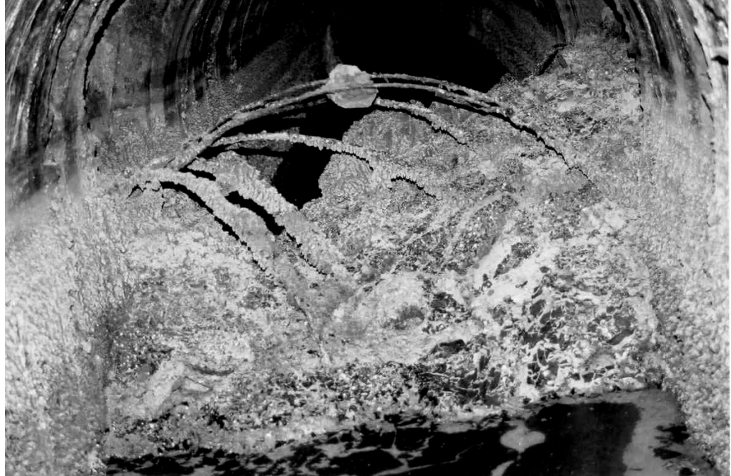
Figure 2.2: View inside Harvey Drift (representing Discharge No 1 at Bowden Close) showing roof collapse into workings.
